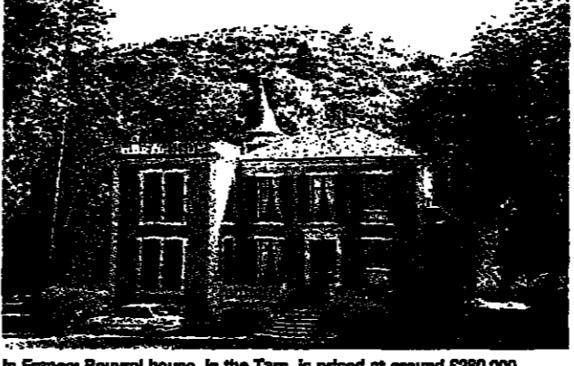
In France: Bouyrol house, in the Tarn, is priced at around £280,000
